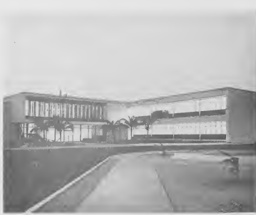
WITH LIGHTS blazing in the early dusk, the new building makes a fine appearance. CU LUZnan cendi den aranan tempran di atardi, e edificio nobo ta haci un aparencia bonita.
